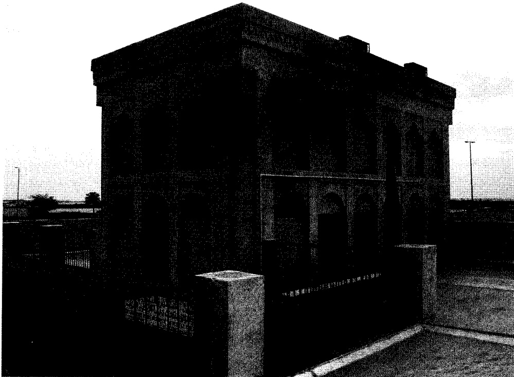
Plate 9: Bayt al-Muraykhî, Dalmâ. Exterior of the upper storey room: view from the NE.
