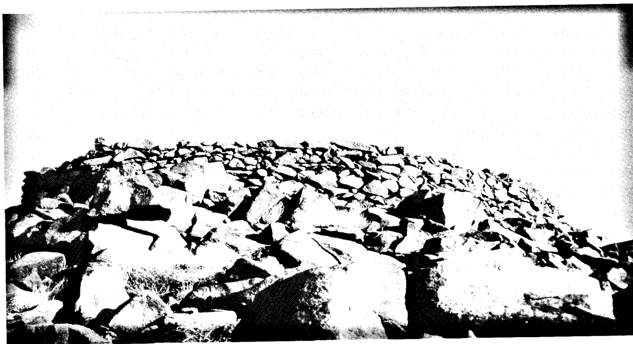
Plate 2: The curtain wall on the west side of the husn
